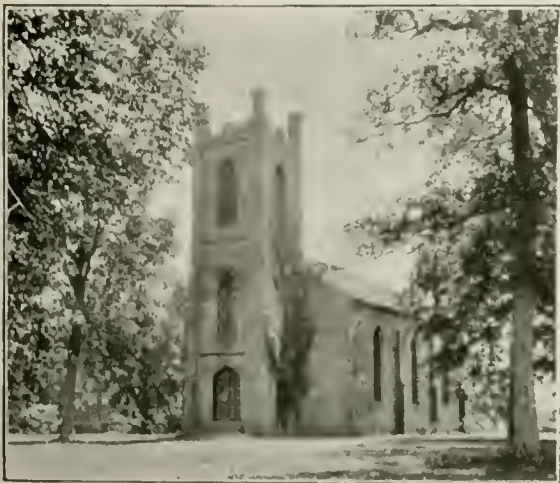
EPISCOPAL CHURCH AT ASHWOOD, TENN.,
